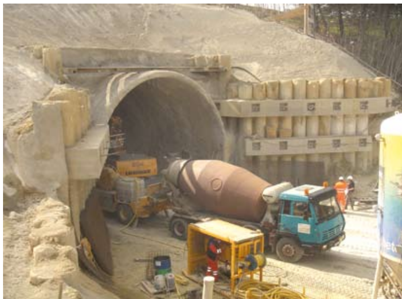
Fig. 7 Support of eastern precut with bored piles and prestressed anchors.
