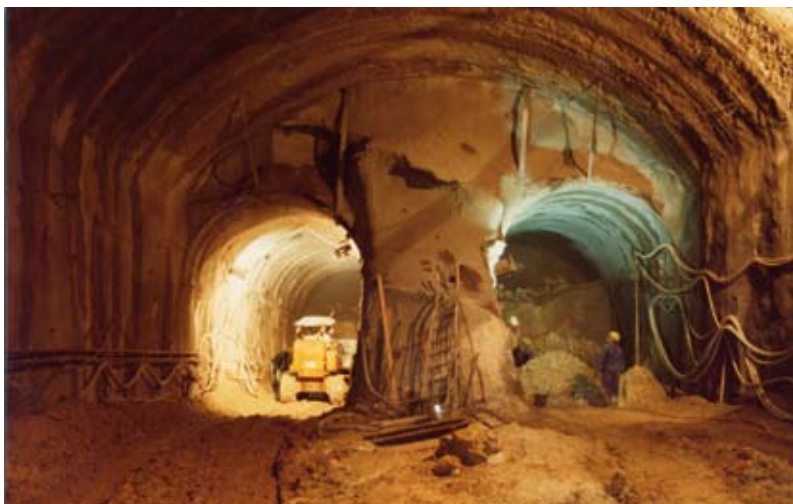
Fig. 4 Side drift excavation, station 50, east drive (1).
